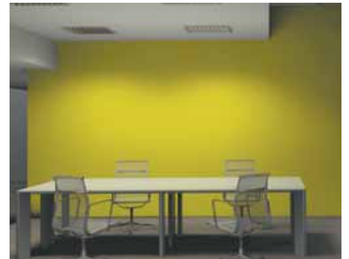
The top render illustrates the performance of a standard recessed 600x600 4x18W T8 module.
